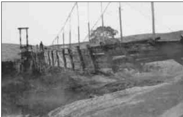
Sandford Suspension Bridge 1940
