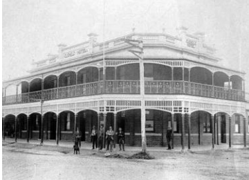
The once impressive verandah of the Glenelg Hotel
